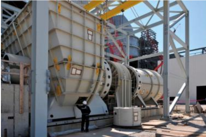
Replacement booster fan on existing foundation
